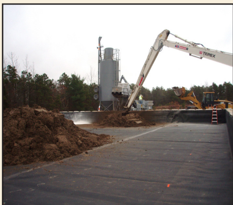
A treatment cell used for bioremediation of explosives contaminated soil excavated from the L Range.
