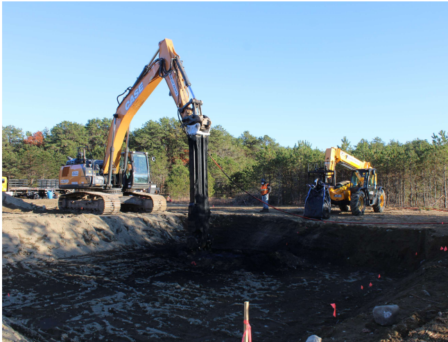
In situ soil mixing of carbon and calcium additives (December 2024)
