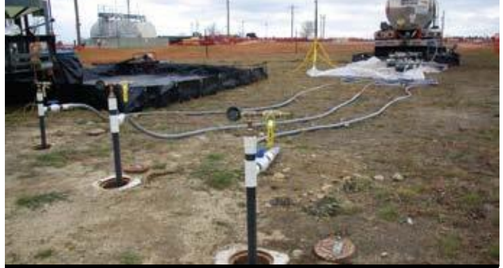
In-situ chemical oxidation operation
